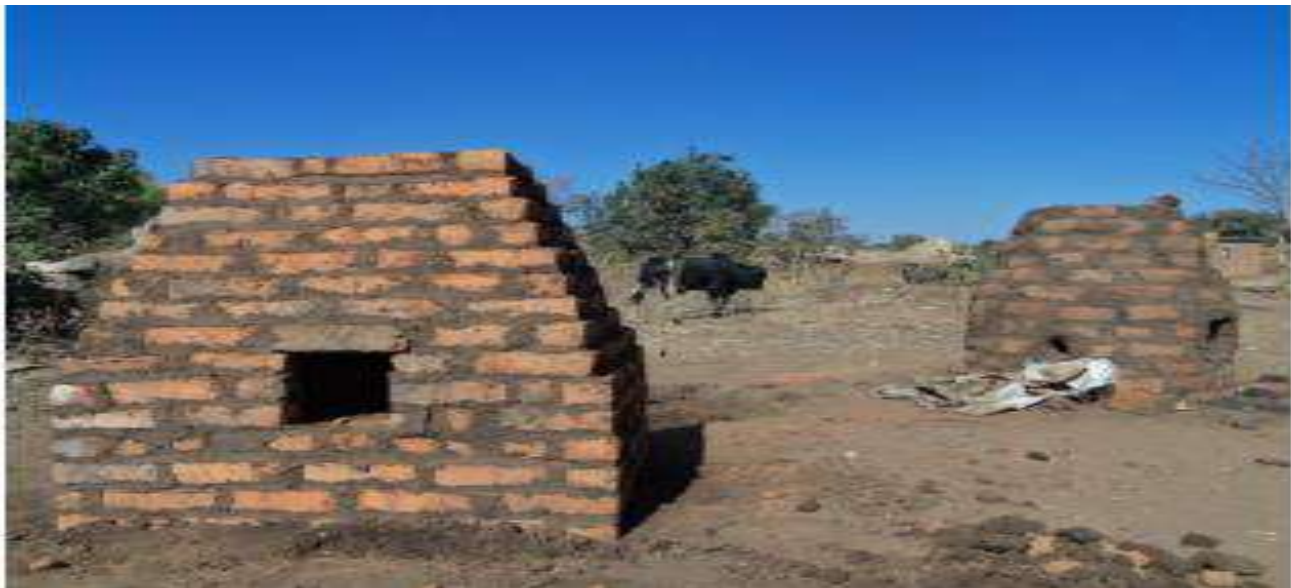
Figure 4: Final kiln (left), African design constructed by community members
